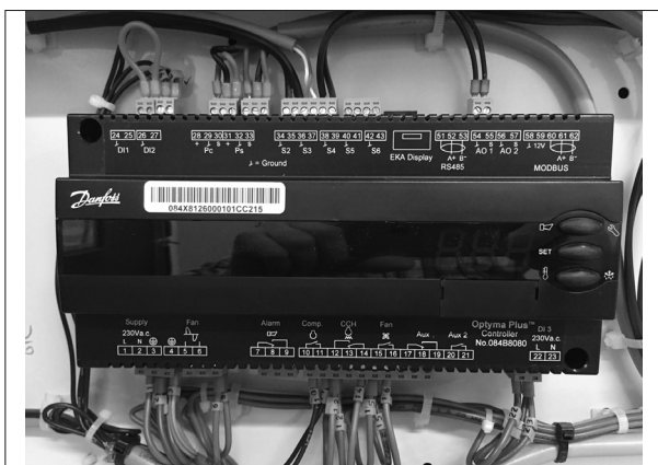
Picture 4 : Normal wiring
