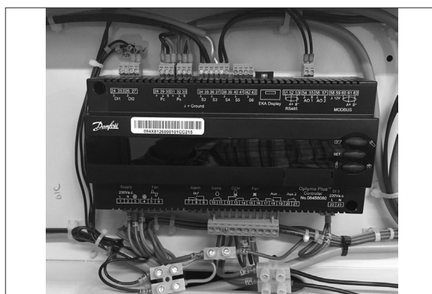
Picture 5 : Temporary wiring
