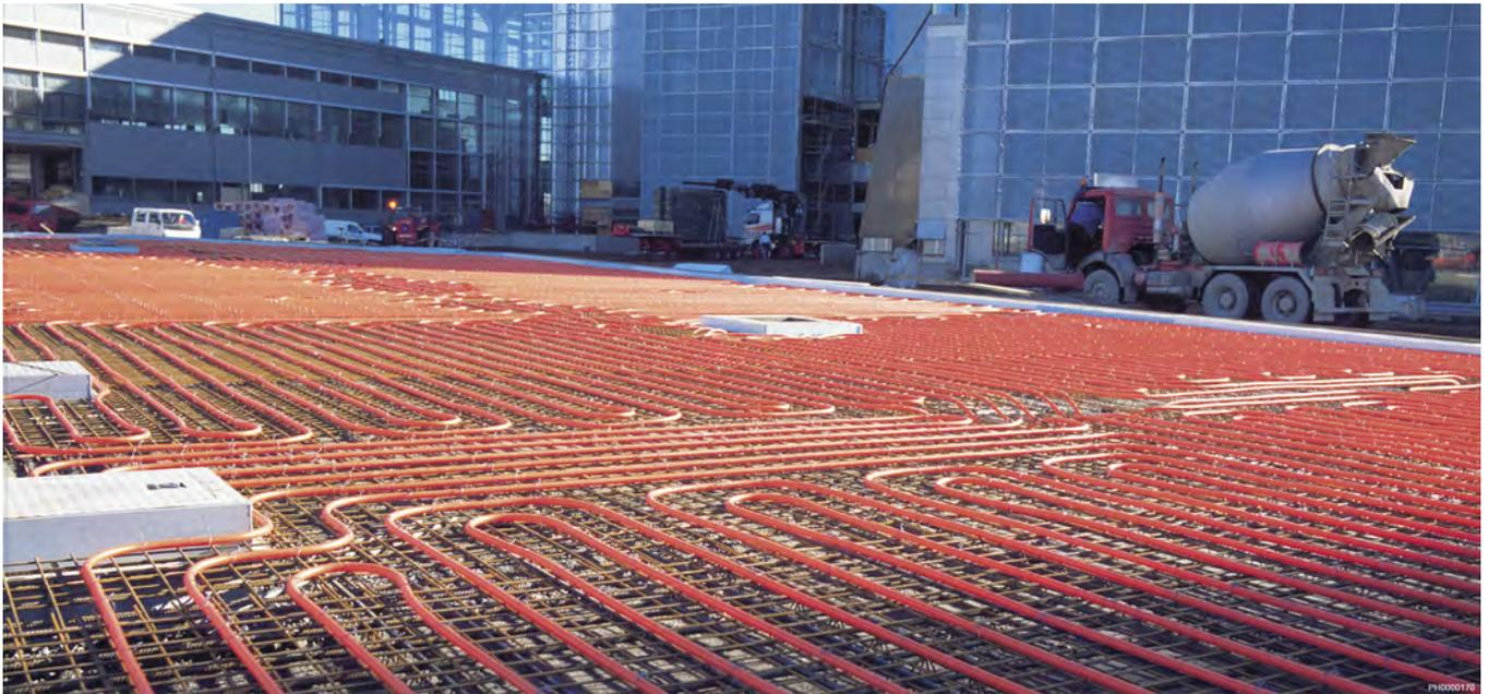
The Uponor Meltaway system is normally installed just underneath the surface layers of the structure. The structural requirements and load-bearing characteristics of such areas must be determined to ensure that predicted loads will not cause the piping to break. The Uponor Meltaway system will not reduce structural requirements.
