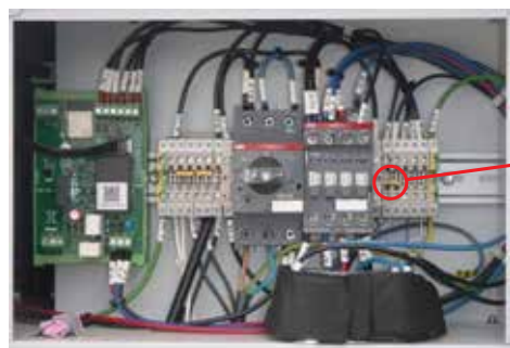
Jumper on slots CNB41 and 43 bridge the digital input DI2. Condensing unit is in pressure control mode.
